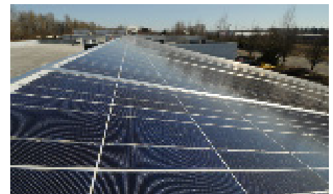
NECA/IBEW solar installation on earth
